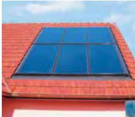
Abb. B.1.6–8 Indachmontage
